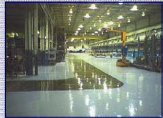
**General Characteristics:** Light stable, high-gloss finish provides light reflectivity. Resists Skydrol®, jet fuels and other industrial chemicals. Provides a high degree of resistance to tire staining. Designed to withstand industrial traffic. Complies with VOC regulations for Industrial Maintenance Coatings below 400 g/l (\*excluding SCAQMD, CARB, &OTC)
