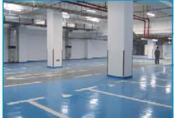
**General Characteristics:** Standard Cure-long working time, Provides a "Breathable" coating to allow transmission of moisture through the coating without failure. 7-12 Perms @ 8mils DFT. Seals concrete, protecting against dirt and spills, Resists staining and minor chemical spills of cleaning and industrial chemicals, No induction time, Complies with VOC regulations for Industrial Maintenance Coatings in the OTC and CA\* (\*excluding SCAQMD for POLYARMOR® EPOXY 40-120W)
