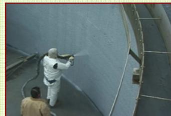
**General Characteristics:** Superior physical properties, 100% solids, highly chemical resistant & abrasion resistant, tough, two part elastomeric spray coating giving rapid and consistent cure in applications ranging from -20°F - over 400°F. Used in demanding installations requiring an elastomeric coating with superior physical properties and very high durability in harsh chemical environments.
