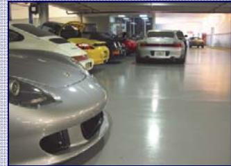
**General Characteristics:** Light stable, high-gloss finish provides light reflectivity, Resists Skydrol®, jet fuels and other industrial chemicals, Designed to withstand industrial traffic. Optional High Wear additive adds 2 times floor life over standard urethanes and adds 4 times floor life over epoxies, Complies with VOC regulations for Industrial Maintenance Coatings in the OTC & CA
