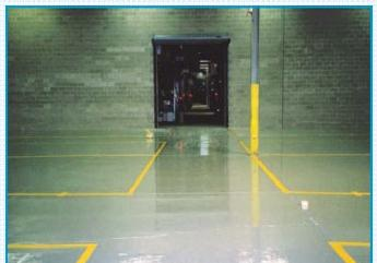
**General Characteristics:** Low viscosity 100% solids fast cure resin, Excellent impact and abrasion resistance, Seals concrete, protecting against chemical spills from many concentrated aromatic & hydrocarbon solvents, inorganic & organic acids, and caustics, Super hard "Tile Like" Semi-Gloss finish, Complies with VOC regulations for Industrial Maintenance Coatings in the OTC and CA.
