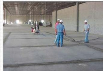
**General Characteristics:** Odorless, Rapid cure in minutes, Excellent impact and abrasion resistance, Flexible, 600% elongation, Remains flexible in cold environments, Resists hot water dumping up to 250°F, High chemical resistance - Resists staining and major chemical spills of cleaning and industrial chemicals, Meets USDA requirements, Complies with VOC regulations for Industrial Maintenance Coatings in the OTC and CA.
