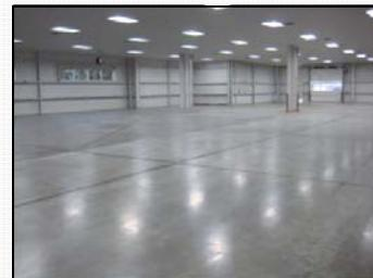
**General Characteristics:** Low Odor, High chemical resistance, Excellent impact and abrasion resistance, Flexible, 600% elongation, Remains flexible, Resists hot water dumping up to 200°F, Resists staining and major chemical spills of cleaning and industrial chemicals, Meets USDA requirements, Complies with VOC regulations for Industrial Maintenance Coatings in the OTC and CA.
