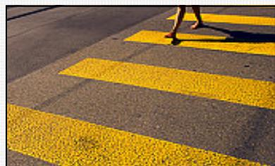
**General Characteristics:** Highly cross-linked plural component polyurea system. Applied in highway marking applications. Aliphatic—extremely color stable under the influence of prolonged UV exposure.
