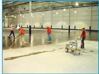
**General Characteristics:** Fast Cure- 2 times faster dry time over standard water borne and standard epoxy systems. Provides a "Breathable" coating to allow transmission of moisture through the coating without failure. 7-12 Perms @ 8mils DFT. Seals concrete, protecting against dirt and spills, Resists staining and minor chemical spills of cleaning and industrial chemicals, No induction time, Complies with VOC regulations for Industrial Maintenance Coatings in the OTC and CA
