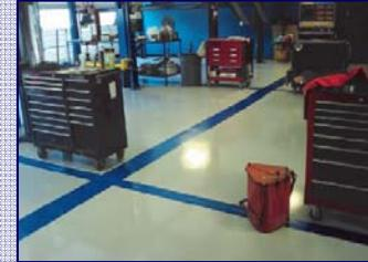
**General Characteristics:** Light stable, high-gloss finish provides light reflectivity, Resists Skydrol®, jet fuels and other industrial chemicals, Designed to withstand industrial traffic. Optional High Wear additive adds 2 times floor life over standard urethanes and adds 4 times floor life over epoxies, Complies with VOC regulations for Industrial Maintenance Coatings in the OTC & CA\* (\*excluding SCAGMD)
